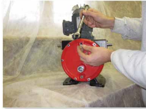
Figure 28: Installation of Pump Vent Plug
